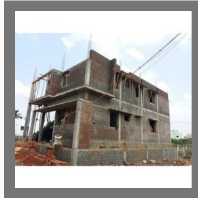
House Construction Service
