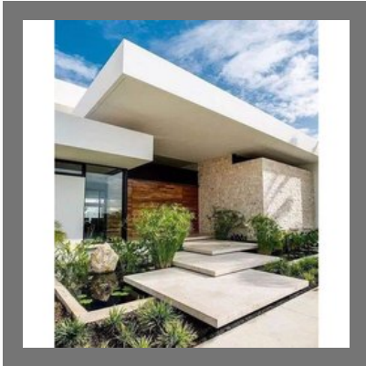
Residential Construction Service
