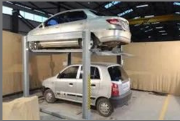
Electromechanical Stack Car Parking
