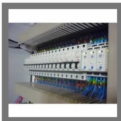
Commercial Electrical Wiring Work
