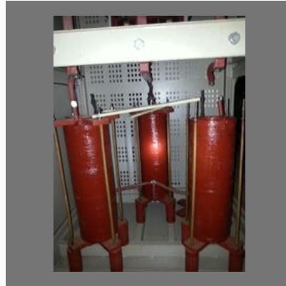
Motor Starting Reactors
