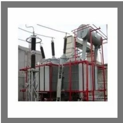
High And Medium Velocity Water Spray System
