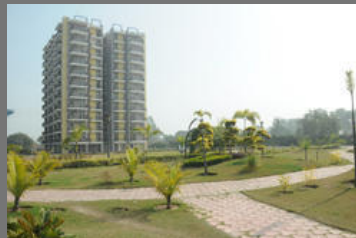
Towers Building Construction Services
