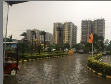
Towers Building Construction Services
