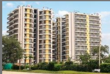
Towers Building Construction Services
