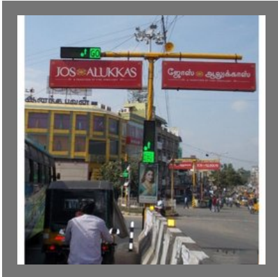
LED Traffic Signal Light
