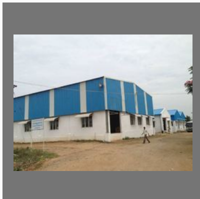
Saredon Steel Buildings
