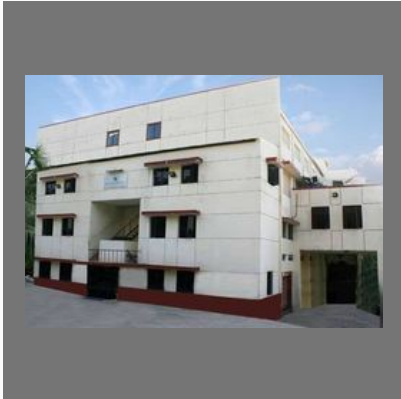
Office Building Construction
