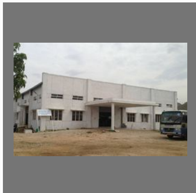
Industrial Building Construction
