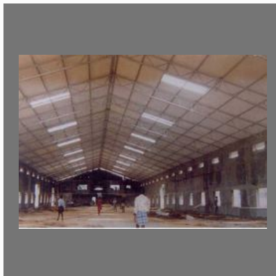
Industrial Building Construction Project
