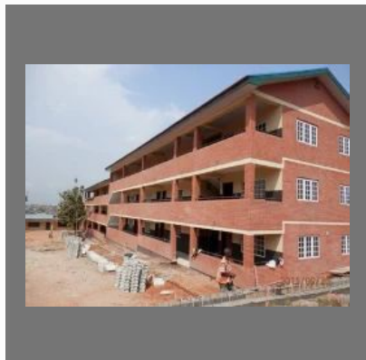
Concrete School Building Construction Service
