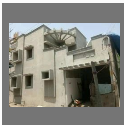
Hotel Construction Service
