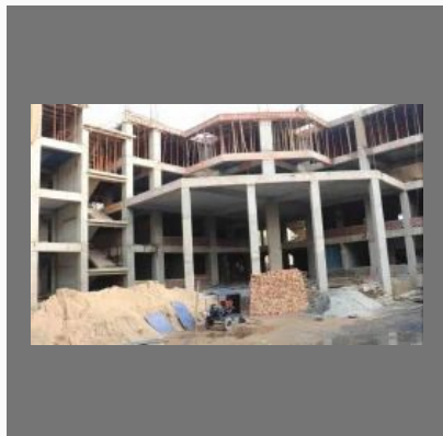
Hospital Construction Service
