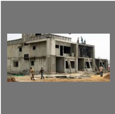
Office Construction Service
