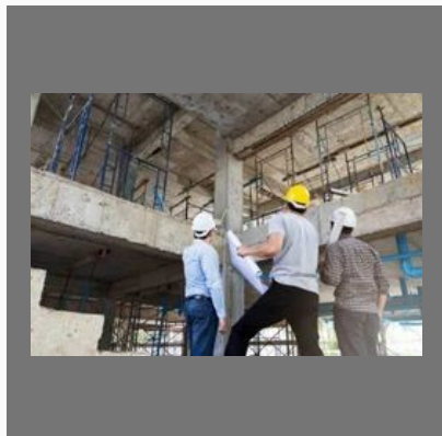
Luxury Villas Construction Service
