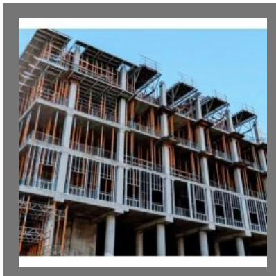
Commercial Building Construction Services
