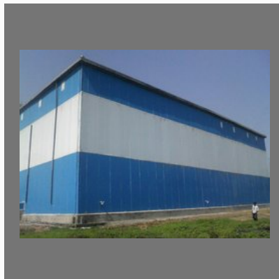
Cold Storage Insulation Service
