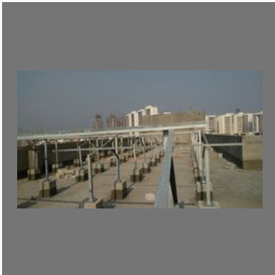
Design And Supply Of Gi Solar Structure
