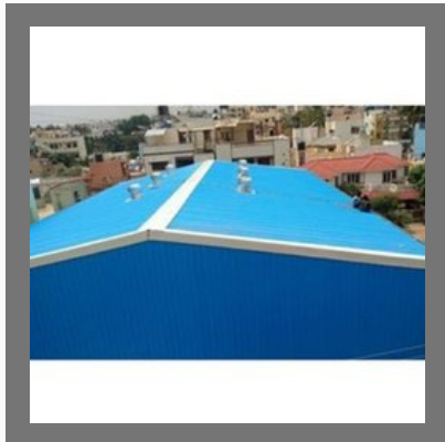
SS Factory Roofing Shed
