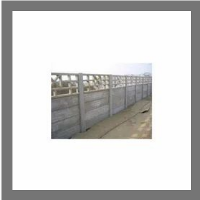
RCC Compound Wall
