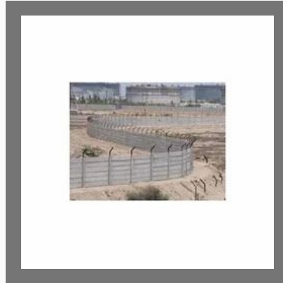
RCC Cement Compound Wall
