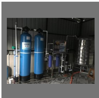
RO Water Purifiers AMC Repairing Services
