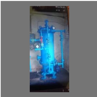
Water Pump Motor Repairing Services
