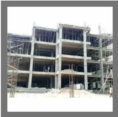
Hospital Building Construction
