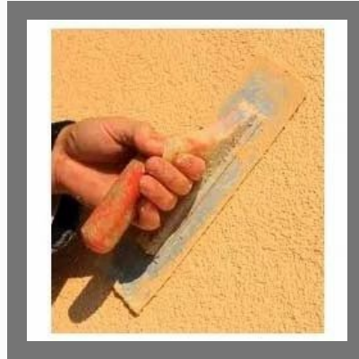
Trowel Finish Painting Service
