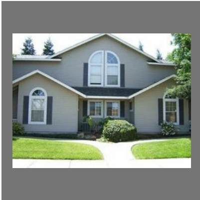
Exterior Paint Project
