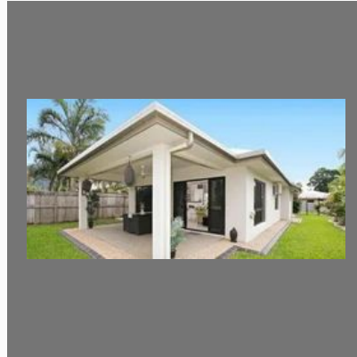
Exterior Wall Paint Project
