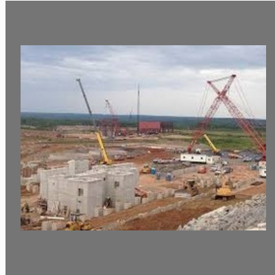
Building Layout Survey
