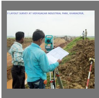
Plotting Demarcation Survey
