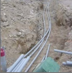
Underground Cable Laying
