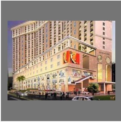
High Street Commercial Shop At Main Road
