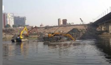
Amphibious Hydraulic Excavator Water Project
