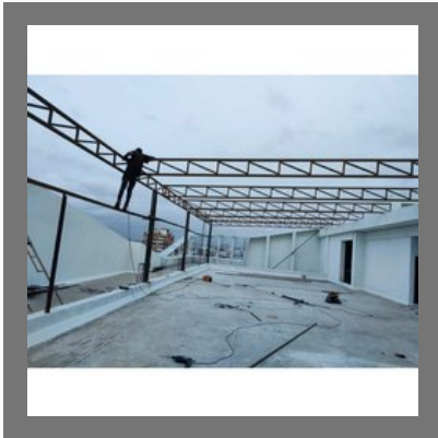
Puff Panel Terrace Roof Structural Fabrication Services
