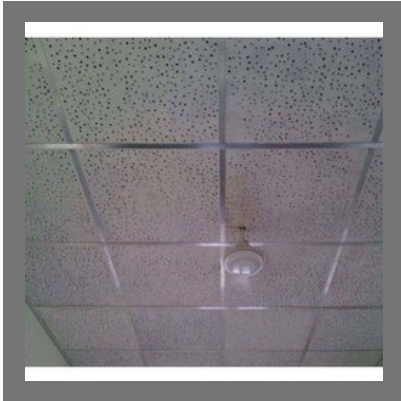
Grid False Ceiling Services
