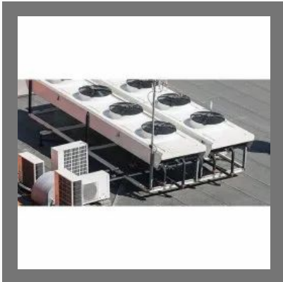
Air Conditioner Maintenance Service
