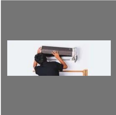
Air Conditioner Installation Service
