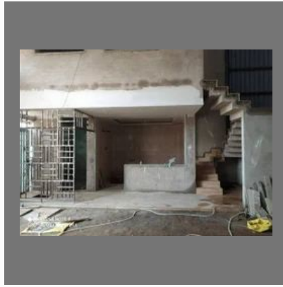
Guest House Construction
