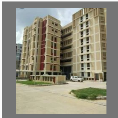
Multistory Residential Building Construction
