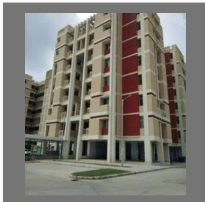
Multistory Building Construction
