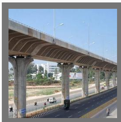
Bridge Inventory Survey
