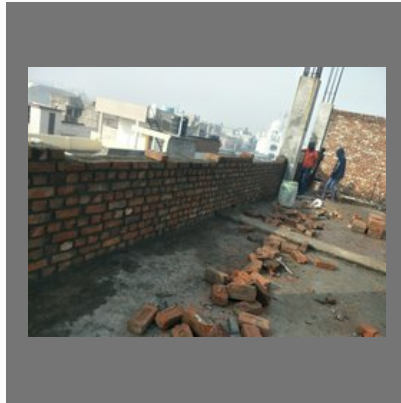
Commercial Construction Work
