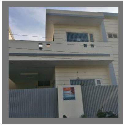
Residential Construction Work
