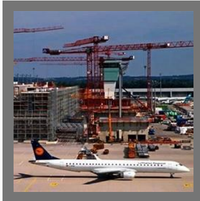
International Airport Construction
