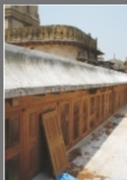
Laxmi Villa Construction
