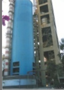
Blending Silo Construction
