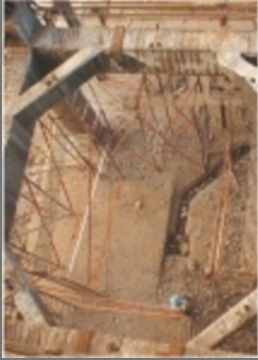
Brine Saturator Construction
