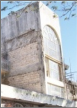
Hotel Building Construction
