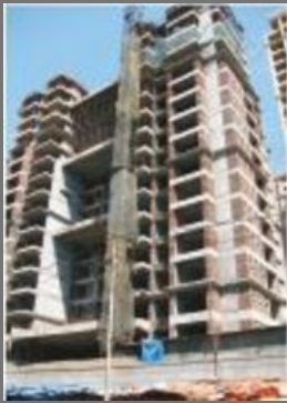
Residential Complex Construction
