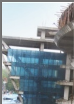
Commercial Complex Construction
