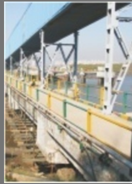
Approach And Jetty Of Bulk Cement Terminal
