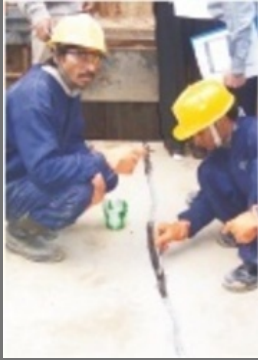
Under Ground Railway Tunnel Construction
