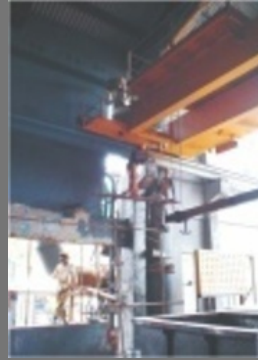
Pickling Plant Construction
