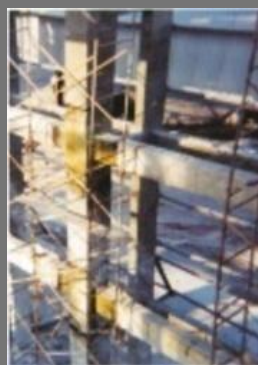
Fertilizer Plant Construction
