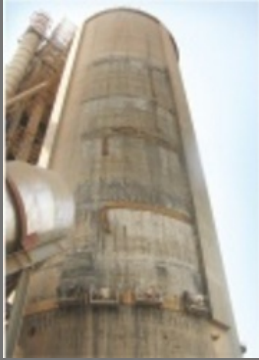
Raw Mill Silo Construction
