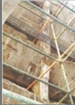
Induced Draft Cooling Tower Construction
