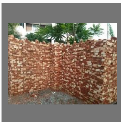
Construction Red Bricks
