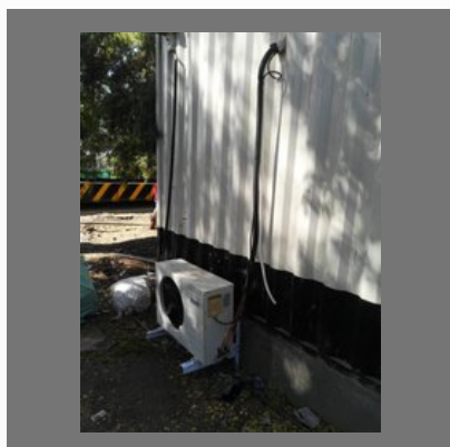
AC Repairing Services
