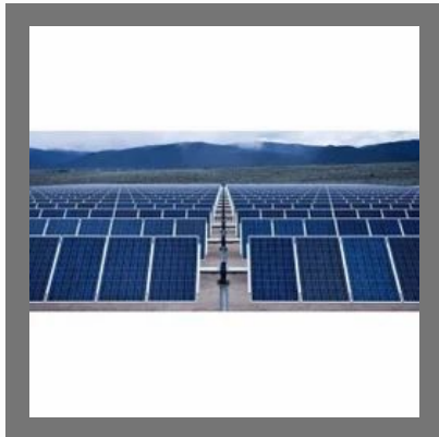
Industrial Solar Power Plants
