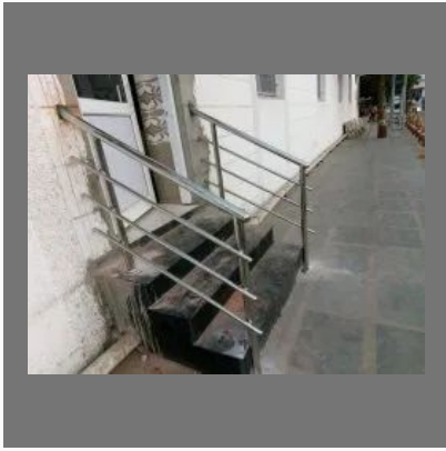
Stainless Steel Railing
