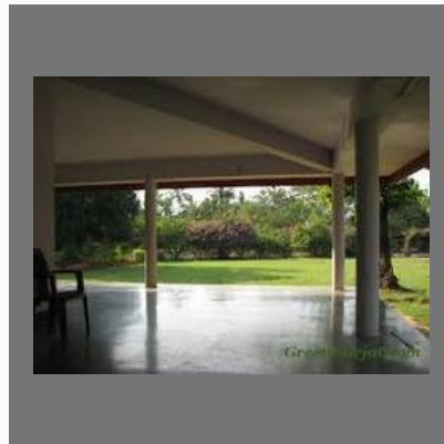
RCC Rooms with Attached Facility Service
