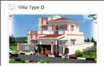
Construction Of Villa Type D
