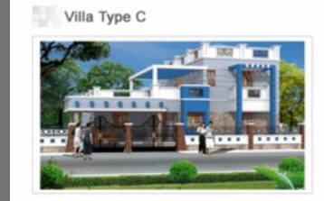
Construction Of Villa Type C
