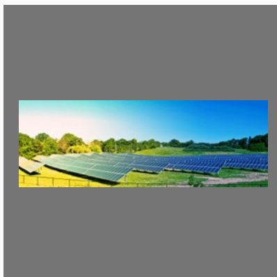
Solar Power Plant
