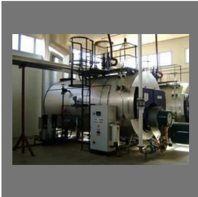
Steam Boiler Erection Service
