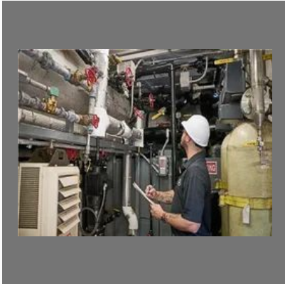
Boiler Repair And Maintenance Services
