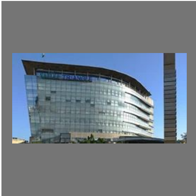
Construction Of Offices
