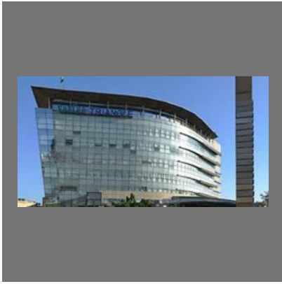
Construction Of Offices
