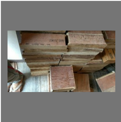
Wooden Switch Board
