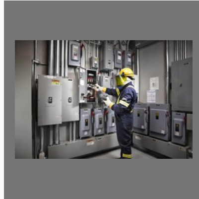
Electrical System Audit
