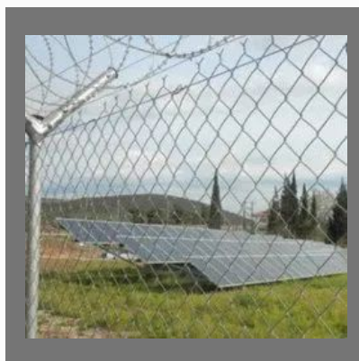
Chain Link Fencing
