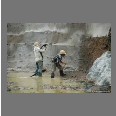
Shotcrete Guniting Work
