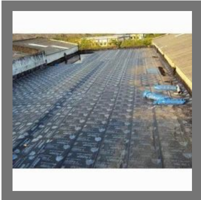
Roof Membrane Waterproofing Service
