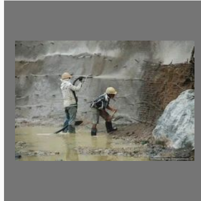
Shotcrete Guniting Service
