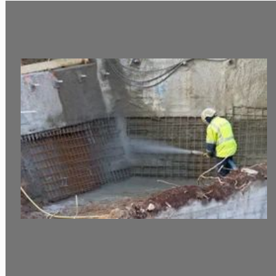
Apartment Shotcrete Guniting Services
