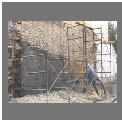
Old Building Guniting
