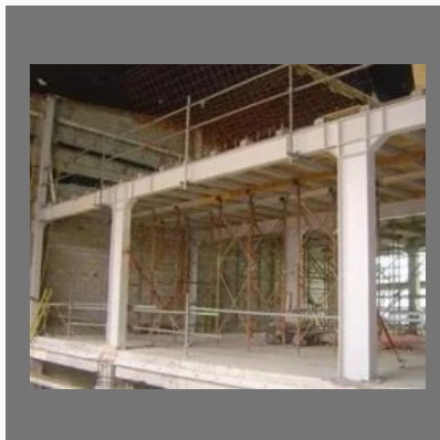
Building Strengthening Work
