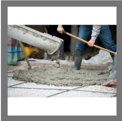
Construction Material Testing
