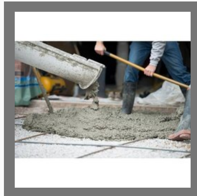
Construction Material Testing
