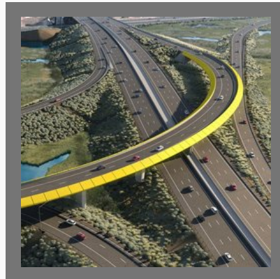
Transportation & Highway Engineering Testing
