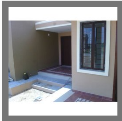
House Construction Service
