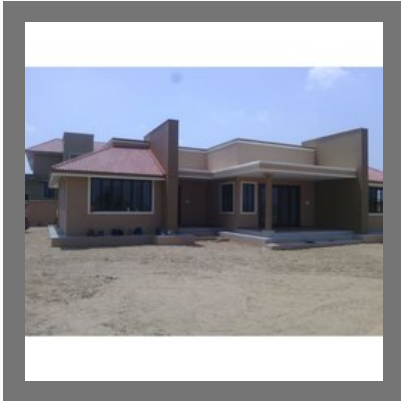
Residential Construction Service
