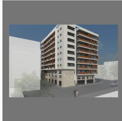
residential building construction
