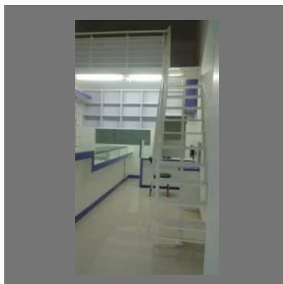
Railing Welding Service
