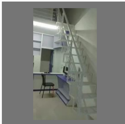
Railing Welding Service
