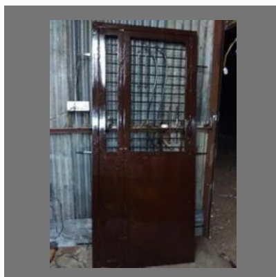
Door Welding Service
