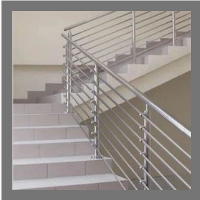
Stainless Steel Railing
