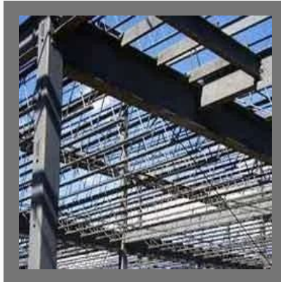
Structural Steel & Fabrication Erection Service
