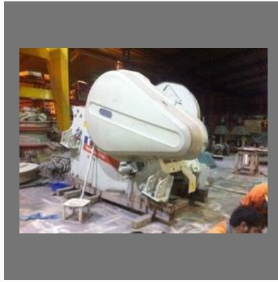
Jaw Crusher Repair
