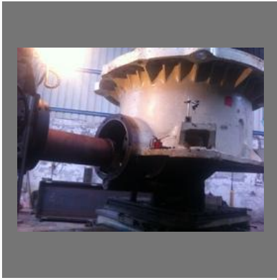
Cone Crusher Repair
