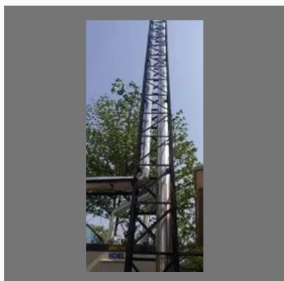
DG Exhaust Stack Structural Assembly With Pipeline
