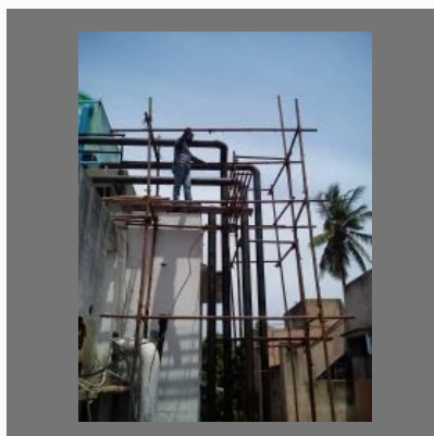
Ms Piping Installation Work
