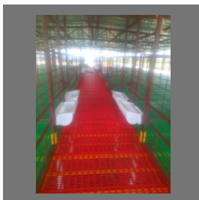
PVC Slated Floor Shed Construction For Sheep And Goat Farming
