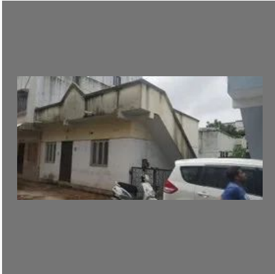
Building Construction Civil Work
