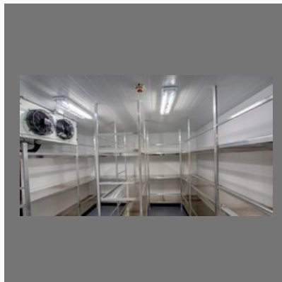
Cold Storage Room
